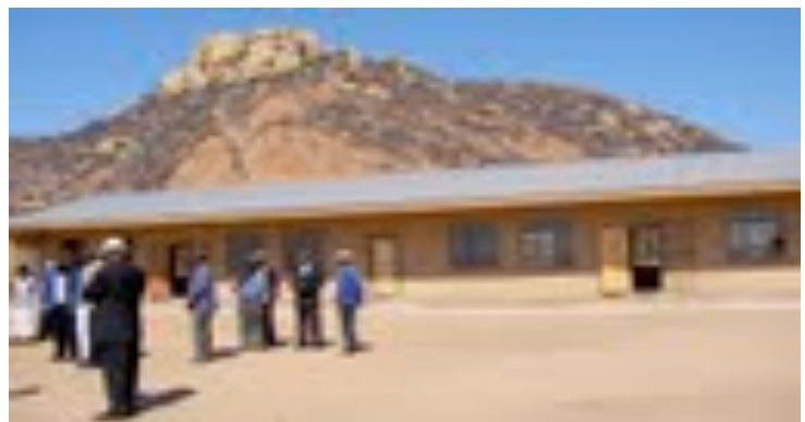
Mogoshi School (K-7 in 4 rooms)
